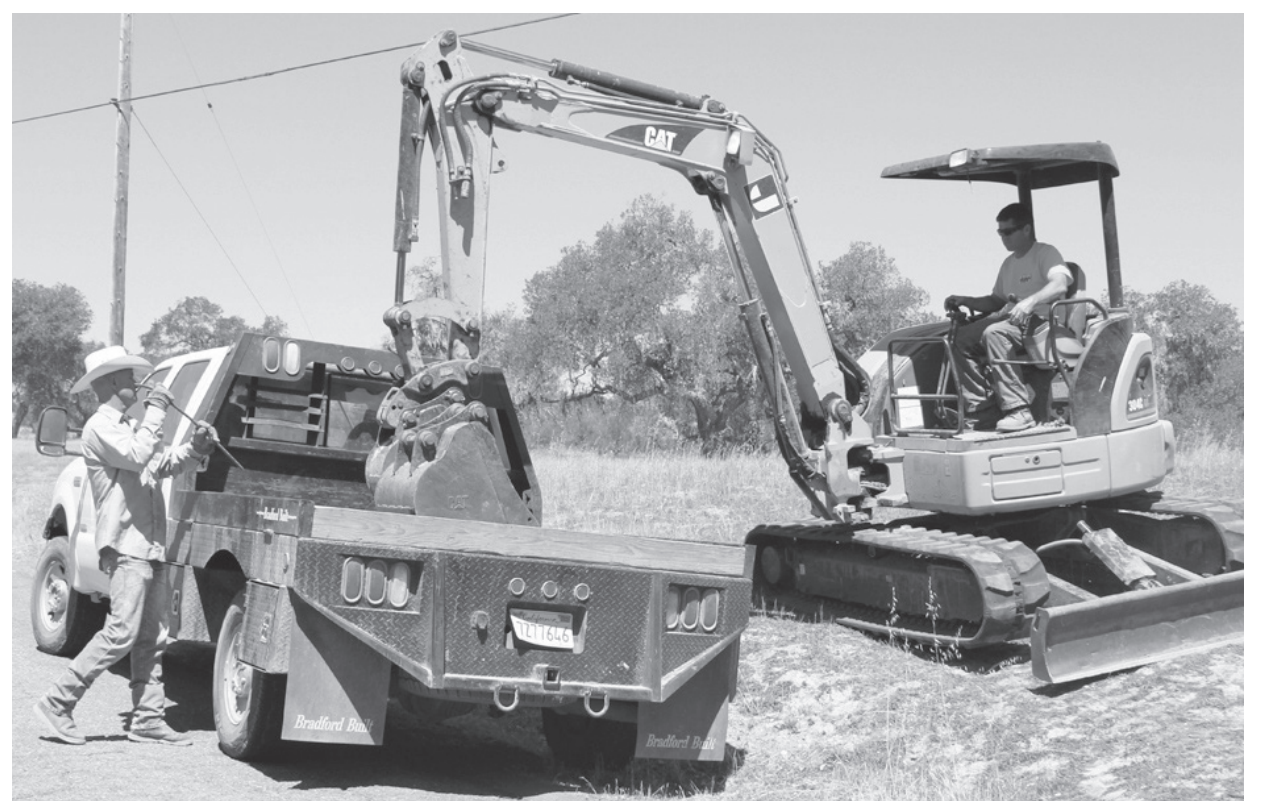
Ranch Manager Randy Campbell gave his full support in the effort to find Kristin Smart. He's shown here helping operator Jim Matthews to switch to a wider bucket on the excavator.
